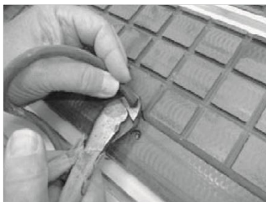
Cutting end of foam rubber gasket
